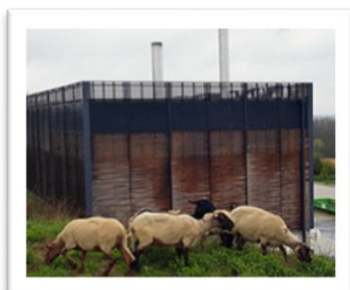
Chaufferie biomasse Auxev
