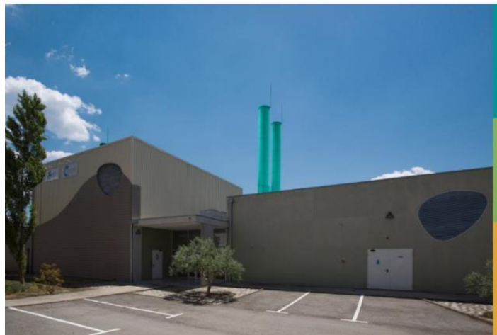
Chaufferie biomasse CALO REM
